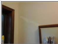
Moderate cracking is evident to wall linings. Periodic maintenance may be required.
