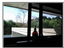
The condition of the windows is generally good. The window catch is missing and requires repair / replacement to restore correct function and security.
