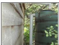
Water tank over flow pipe needs to be connected to the over flow pipe.
