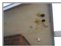
The paint work to the eaves is deteriorating in some areas and maintenance is required.
