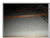
There is no insulation provided to the pitched roof ceiling cavity.
