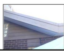
Fascia boards are constructed of timber. The paint work is deteriorating and maintenance is required.
