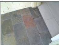
Cracking is evident to some floor tiles. Cracked or damaged floor tiles should be replaced.
