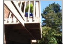
Moderate to severe wood decay is present to the structure. Some repairs or maintenance will be required.
