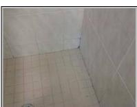
The condition of the splashback tiles is generally good. Some cracked tiles were noted in this area. Rectification may be necessary, contact a floor and wall tiler for rectification.
