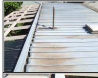
The gutters and downpipes are in good condition. Leaves and debris are present in gutters. These should be cleared to ensure that stormwater is adequately removed from the roof. Note that due to inability to inspect all gutter surfaces due to debris, defects may be present that do not present themselves until gutters are cleaned.
