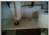
Water staining noted to vanity cabinet. Repairs or maintenance will be required.
