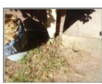
Front right downpipe socket is broken and needs repair to control the stormwater.
