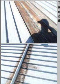
The metal roofing is rusting and requires repairs and rust inhibiting treatment to ensure the roof remains watertight and to limit further deterioration until such time that replacement of the roof sheets is required.
